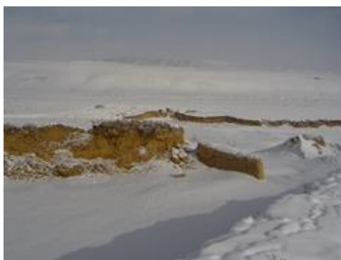
Photo 1: Ground fissures at Xiaoxigou gully mouth
